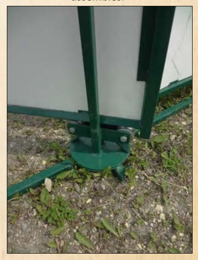
1. Place "swing n slide" door circular plate over top of circular plate that is attached to the straight crowding tub section. (This piece also has the alley entrance included in it.)
